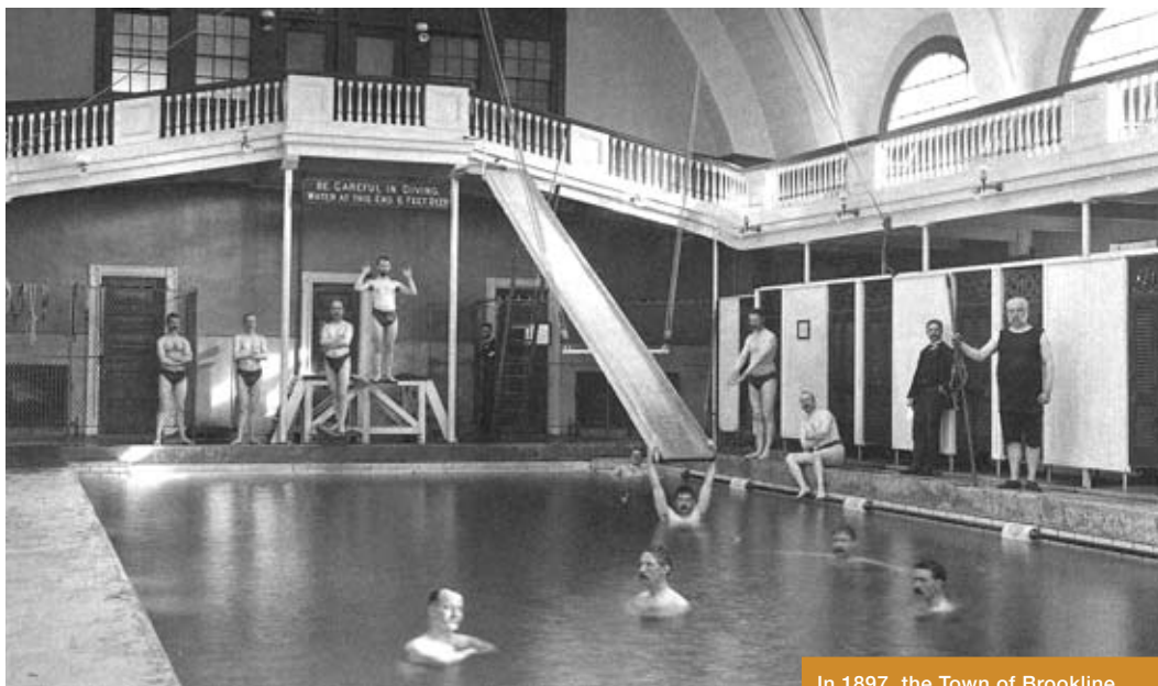
Brookline Preservation Commission
